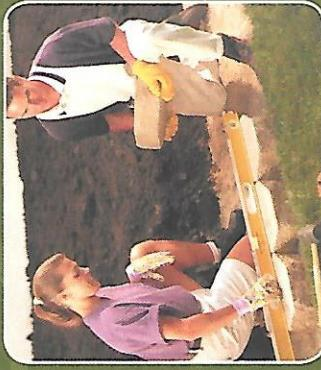
Start by digging a shallow trench 4" deep by 12" wide. Cut through and remove any sod, roots or large rocks. For organic loam soils, dig 4" deeper and add a leveling pad of sand or gravel. Compact and level the soil to receive the first course of Keystone Garden Wall.
