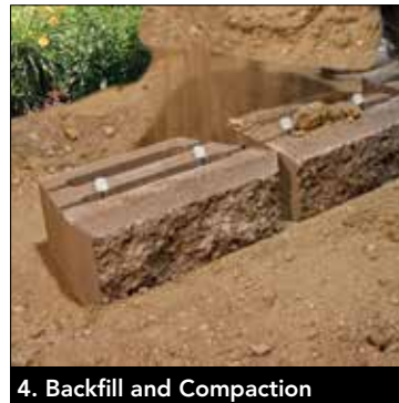
4. Backfill and Compaction
